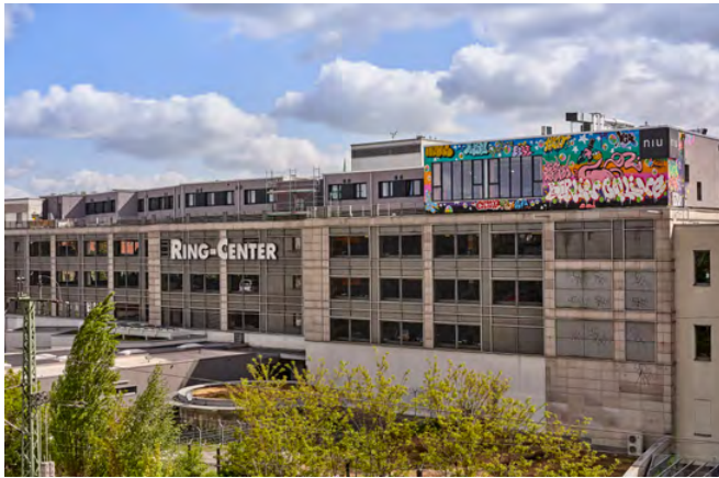
During the course of the expansion of the Ring-Center in Berlin, an NIU hotel was placed on top of the upper parking level using a modular construction method.
